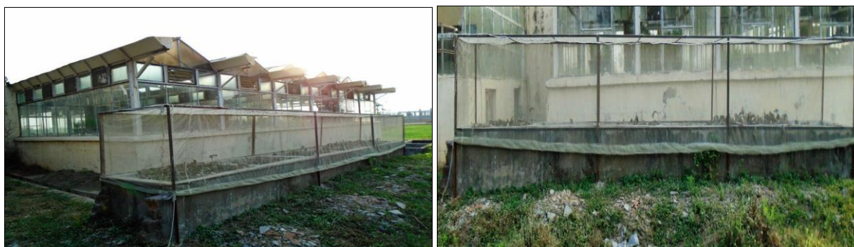
Plate 1: Concrete tanks built to maintain water hyacinth and water hyacinth weevil, N. eichhorniae
