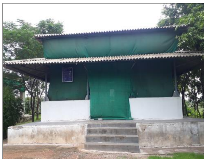
Fig 2: Tubular Structure Grainage House
