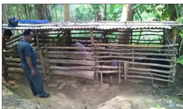
Fig 1: Pigsty made of locally available material with tin roof at Dhalai district
